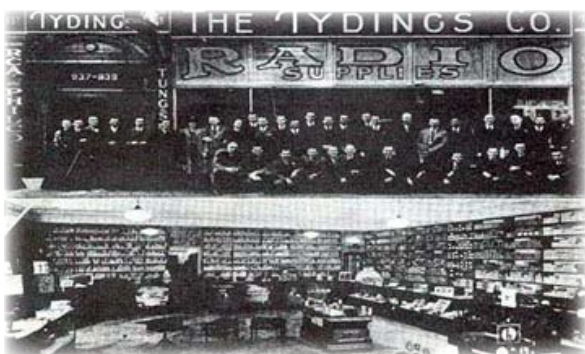
Exterior and Interior Views of The Tydings Co. Circa 1939
