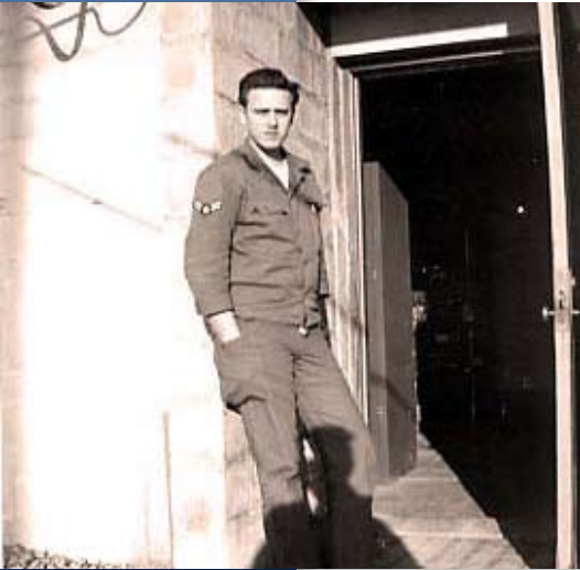
Airman James B. Davis at the Red Head Receiver Building
