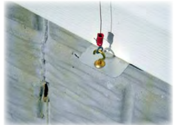
Stealth Antenna Ending at Foundation
