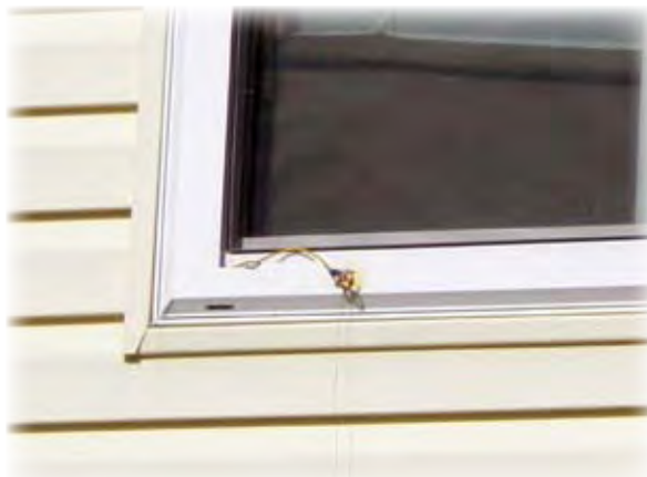
Stealth Antenna Exiting Second Story Window
