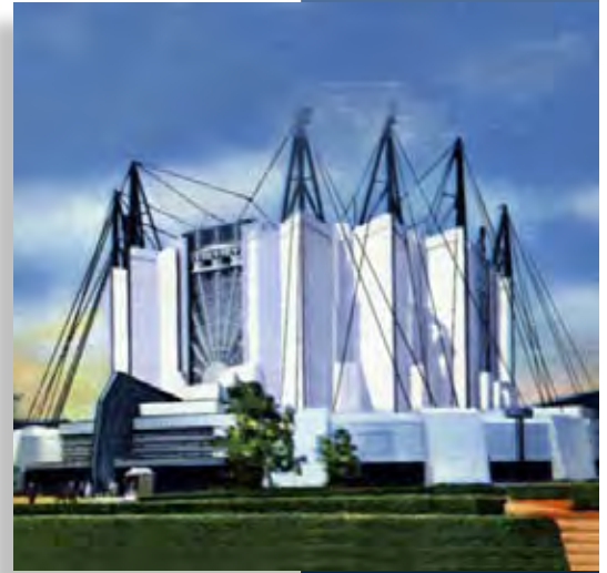
Travel and Transport Building
