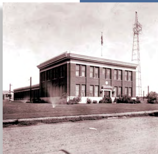
KOA Radio Transmitter Building and Antenna
