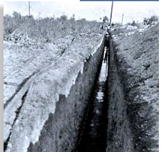
To ensure there was no radiation from wires or cables in the vicinity of the DF, all cables were buried six feet deep.
